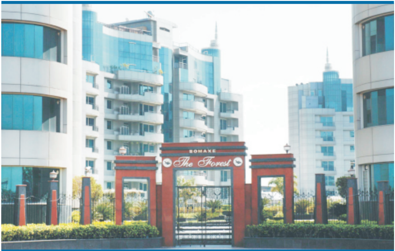
Construction for Omaxe Construction Ltd. The Forest Ultra Luxurious Residential Complex Plot No. 214A, Sector-92, Noida (U.P.)
