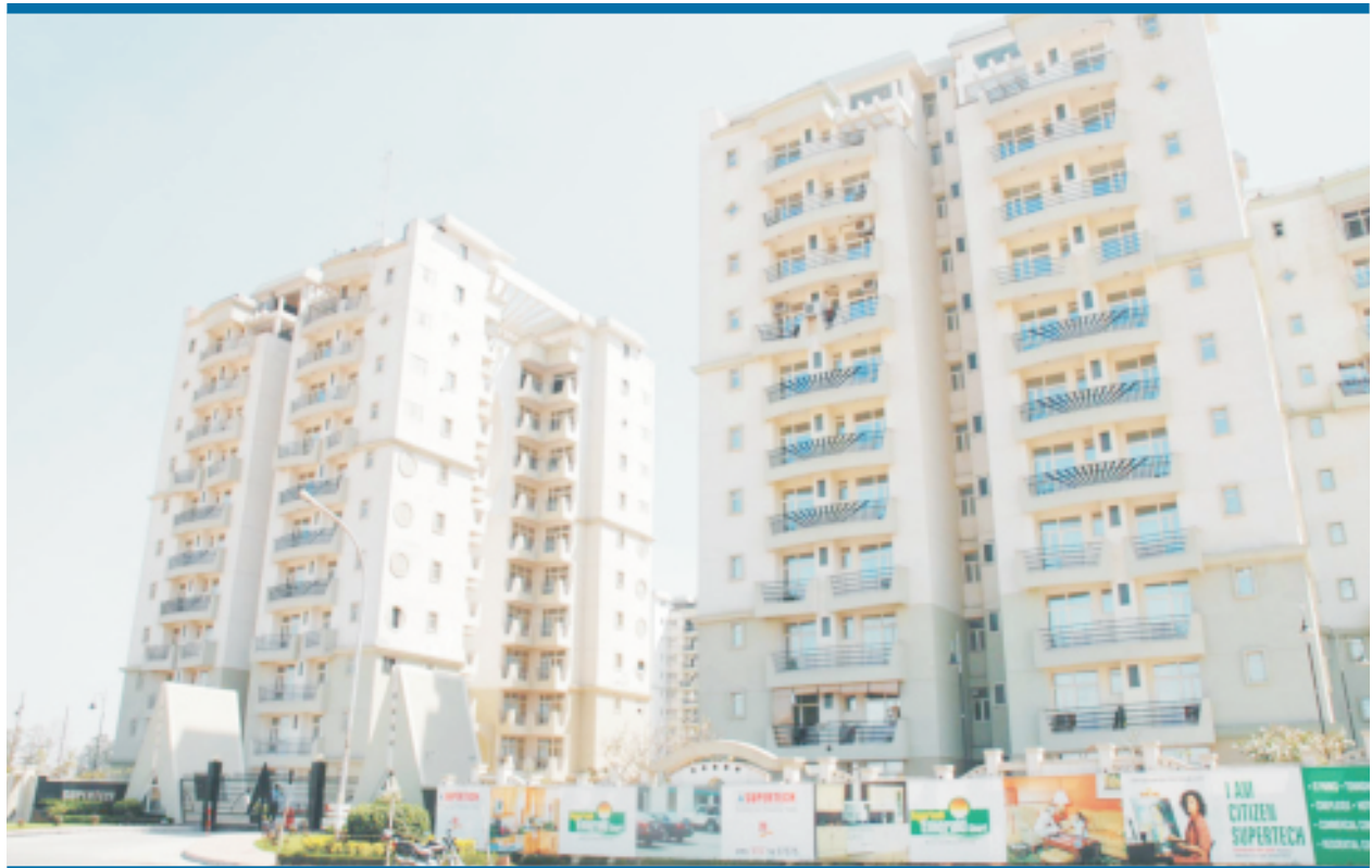
Construction for Supertech Construction P. Ltd. The Emrard Court 130 Flats Residential Building, at Plot No. 04, Sector-93, Noida.
