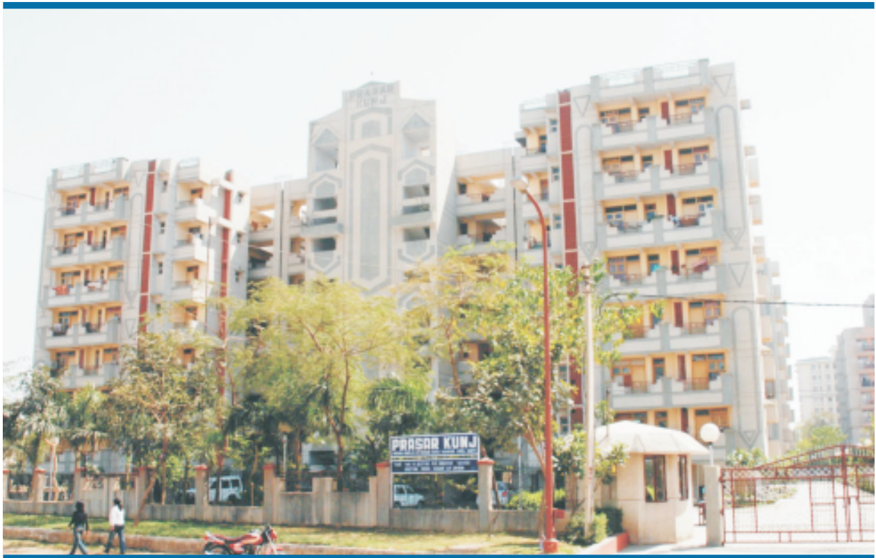
Construction M/S Prasar Kunj Sahkari Awas Samiti Ltd. at Plot No. 08 Sec-Pi. G. N.
