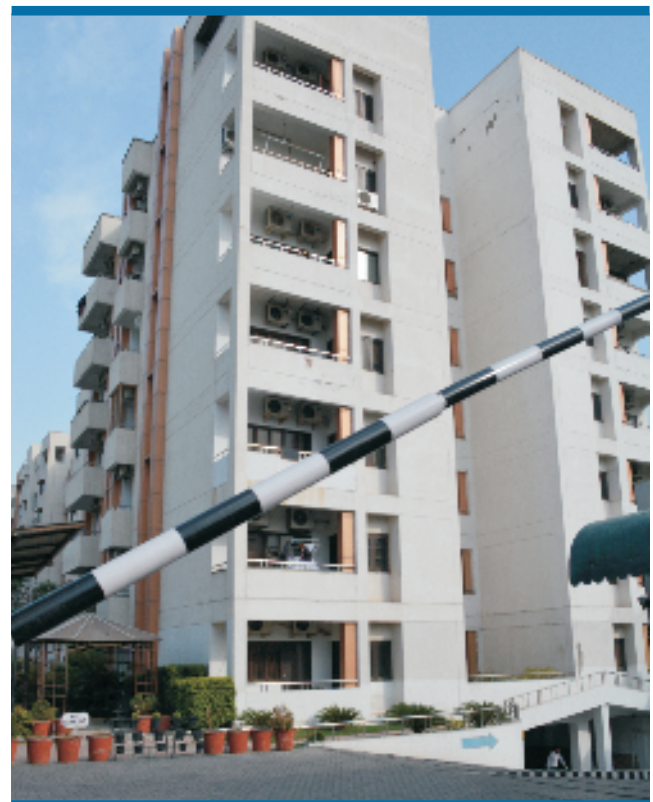
Construction for Group Housing Building Emerald Square at Lajpat Kunj Agra (U.P.) Eminent Infradevelopers Pvt. Ltd.
