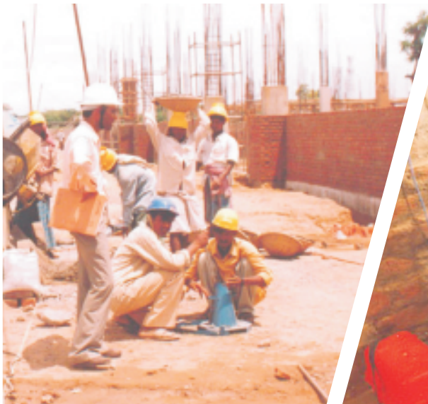
Slump Test
