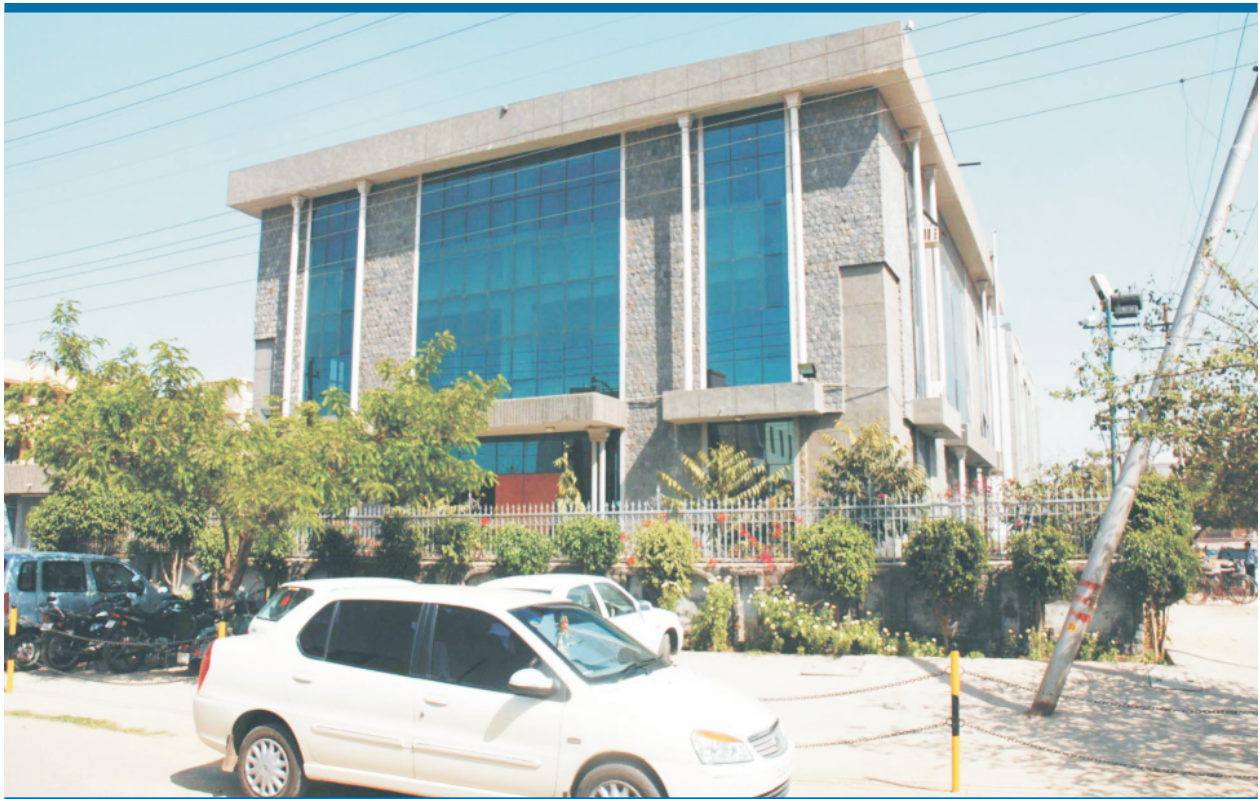
Construction for Mr. Vipin Kumar Jain Factory at Plot No. A-1, Sector-63, Noida
