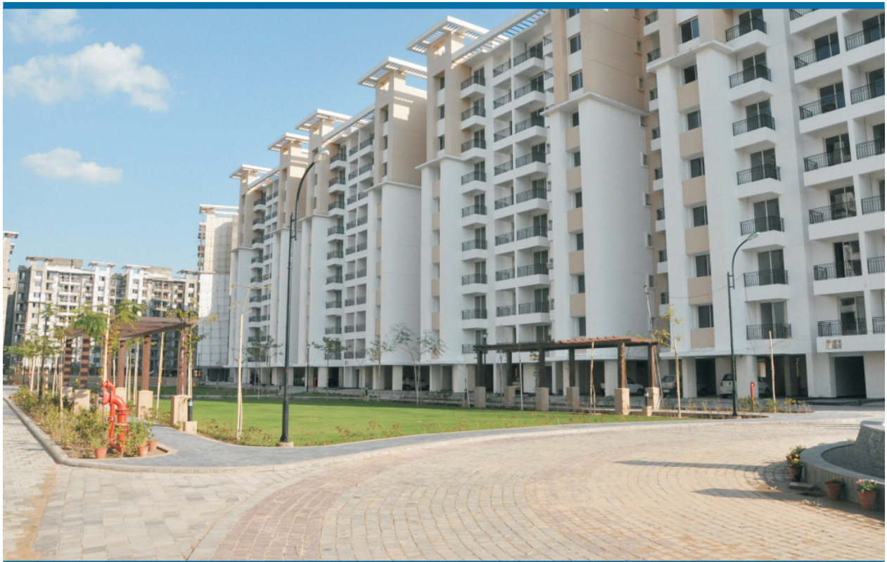
Construction of Urbana Jewels
