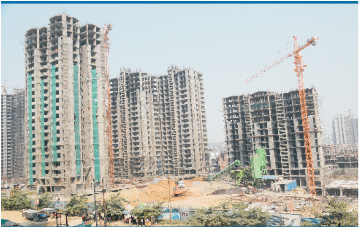
Construction of Samridhi Grand Avenue Noida Extn. Greater Noida
