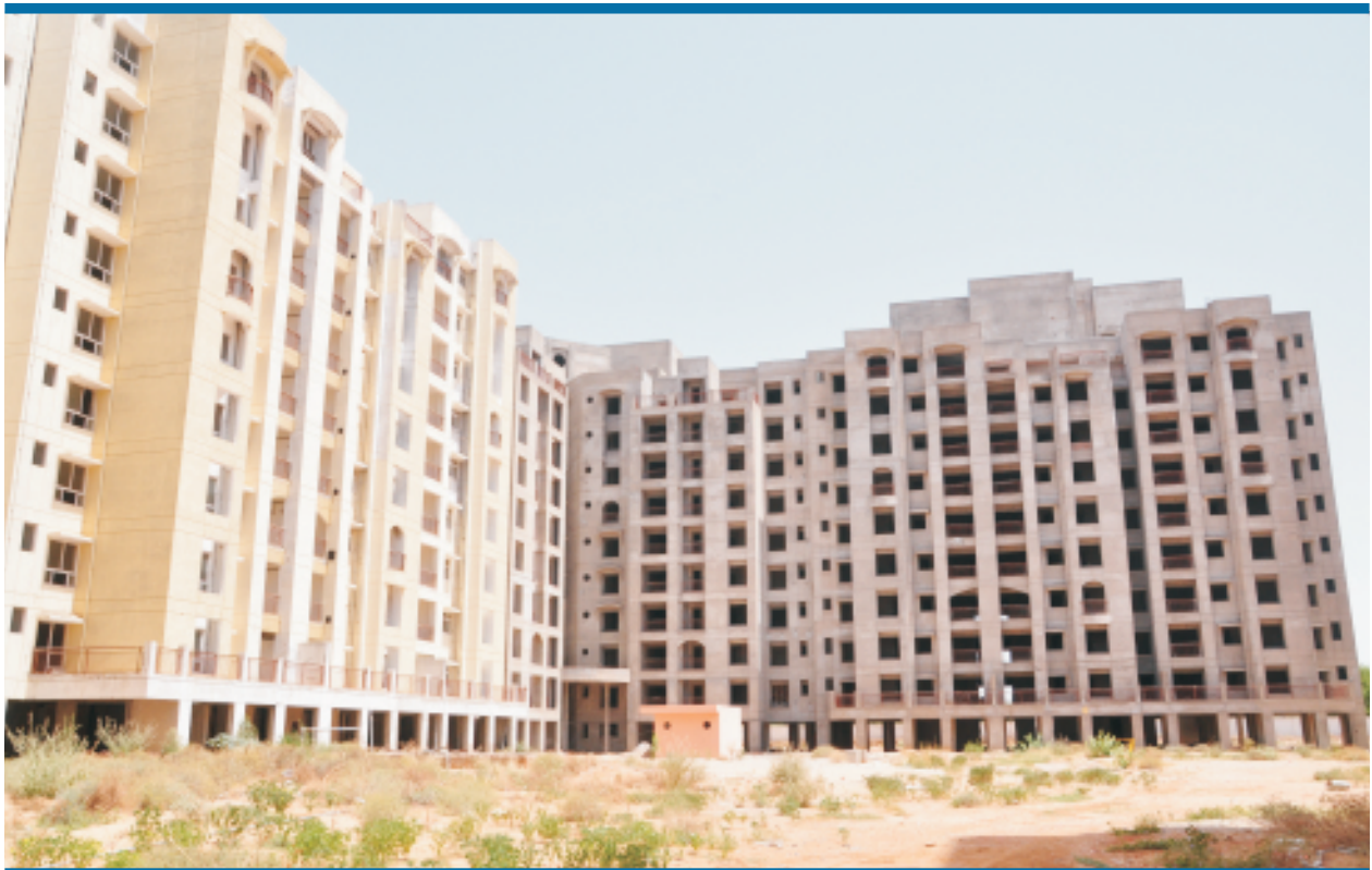
Construction of Sahara Prime City at Jaipur
