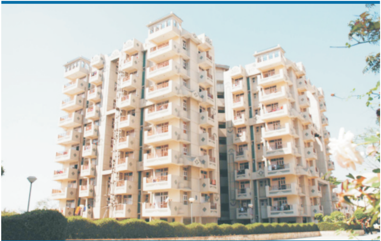
Construction of M/S Khushboo Sahkari Awas Samiti Ltd. at Plot No. 11, Sec-Pi, G. N.
