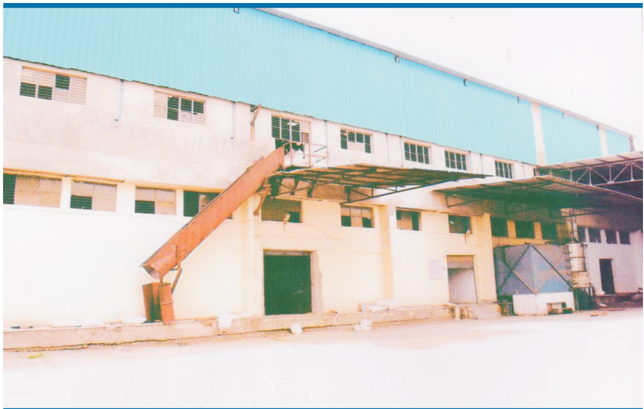
Construction of Suruchi Foods Pvt. Ltd.
