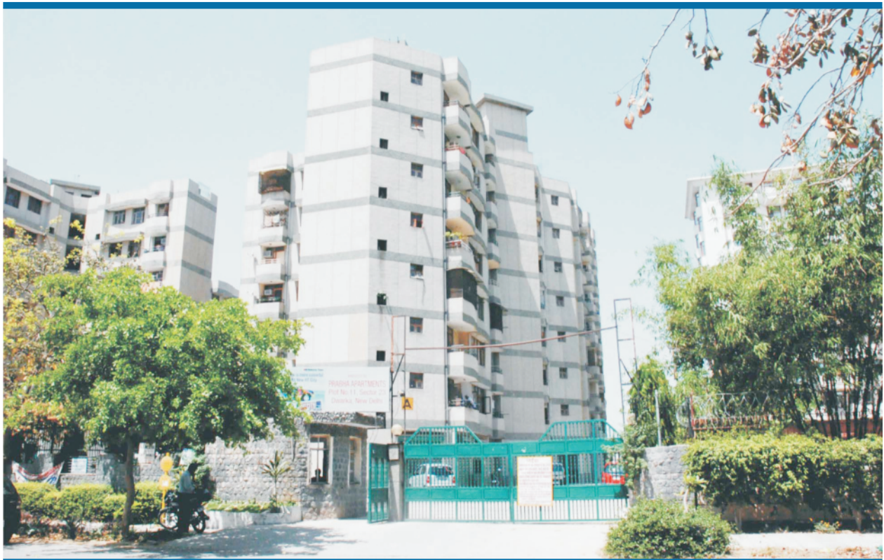
Construction of M/s Prabha Co-op. Group Housing Society Ltd. at Plot No. 11, Sector-23, Pappan Kalan (Dwarka) Delhi.
