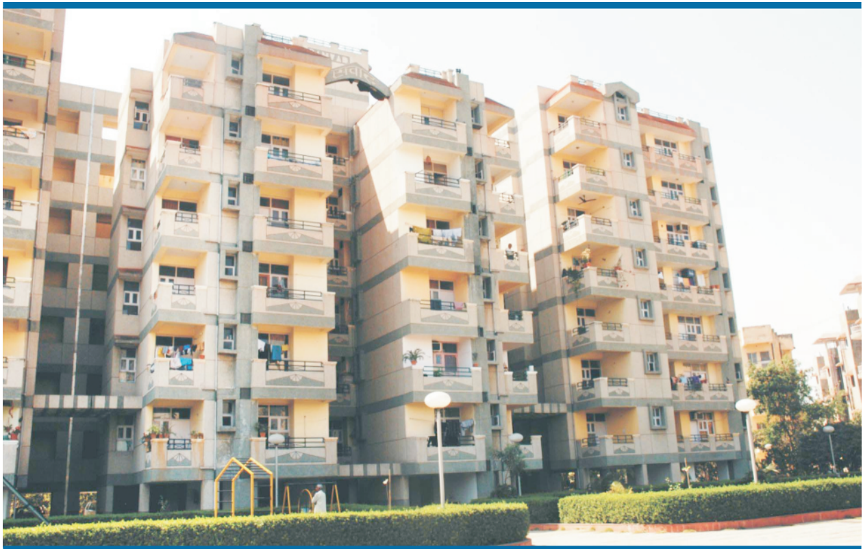
Construction of PTI Co-op. Housing Society LTD at GH-07 Pocket-E, Alpha-I, Greater Noida
